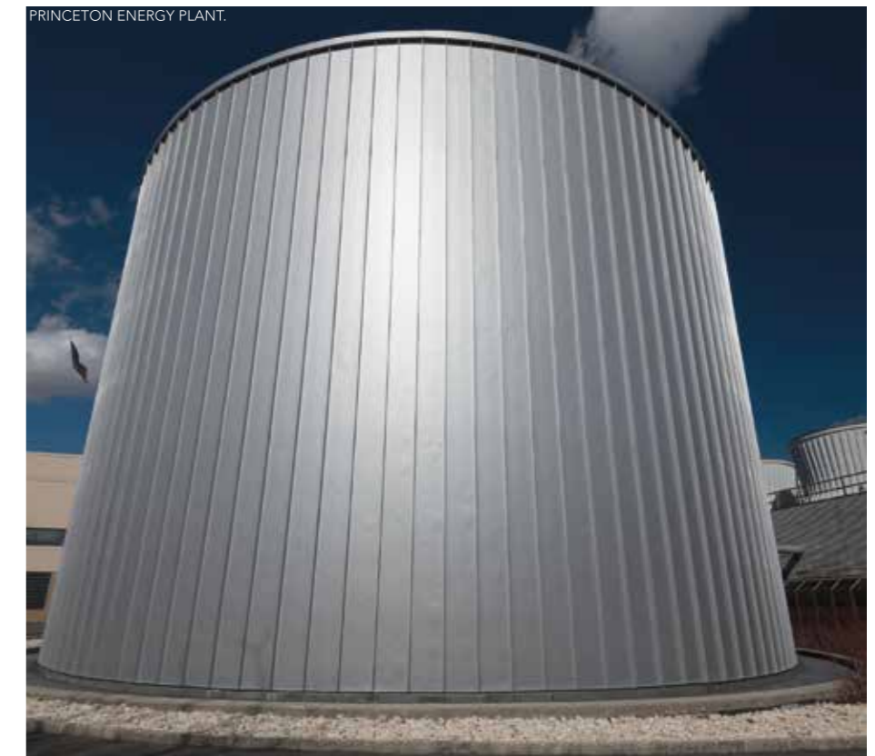
PRINCETON ENERGY PLANT.
