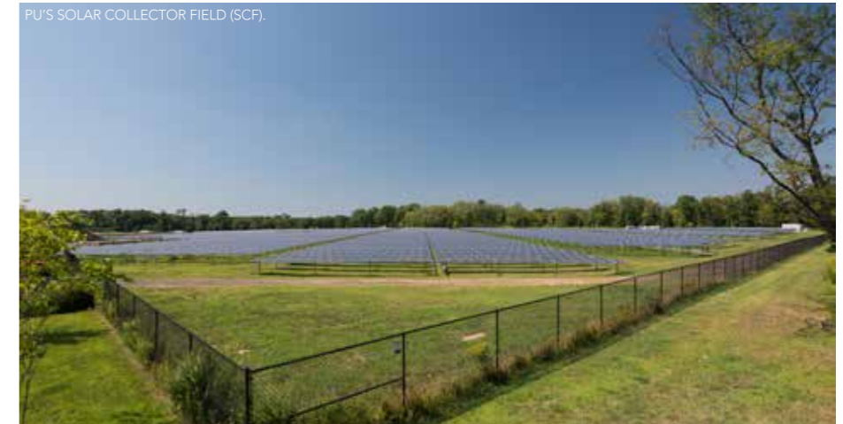
PU'S SOLAR COLLECTOR FIELD (SCF).
